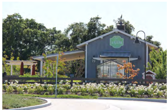
Examples of community buildings, including a clubhouse and a farm activity center.
